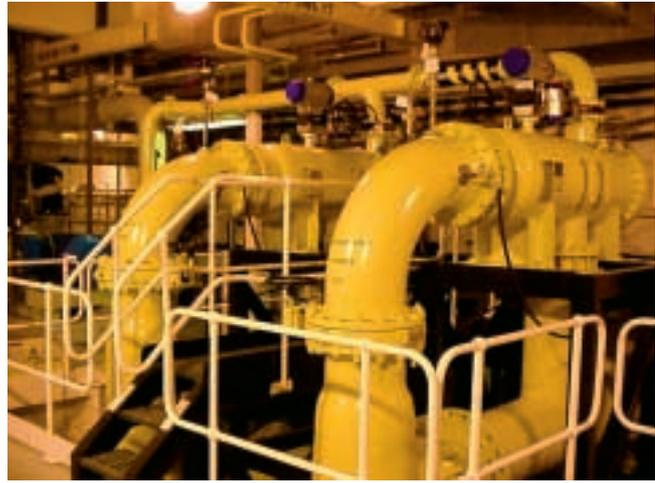
The Alfa Laval ALF filters are mounted horizontally in the seawater piping system.
