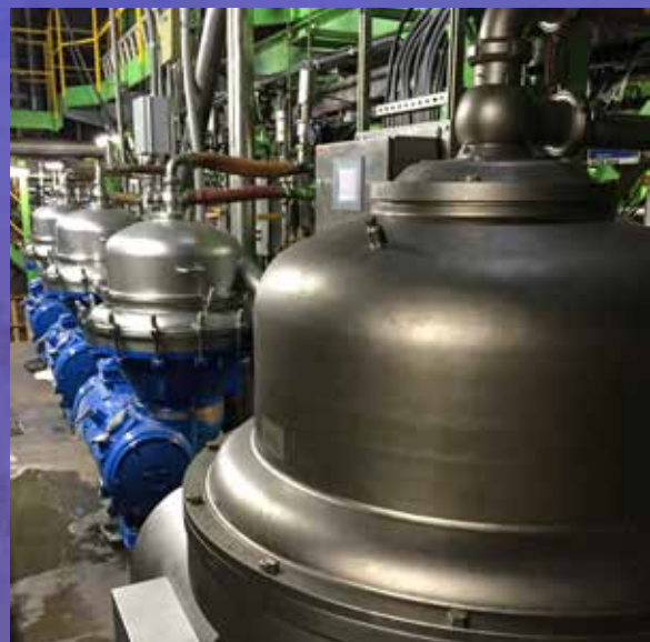
The Alfa Laval skimmer allows Westward Seafoods to reduce oil content in its stick water to less than 0.5%.
