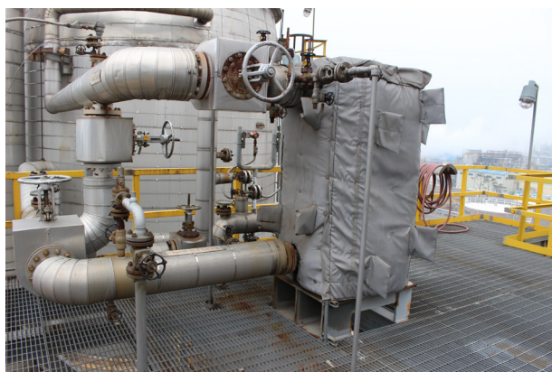
Figure 3. Compabloc installation on a platform.
